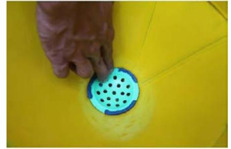
2. Shake all the Drain Pipes to see how sturdy they are. Ensure that there is a slight angle sloping downwards to the drain to let the urine flow easily to the drain without any blockage, at all Drain Pipes.
