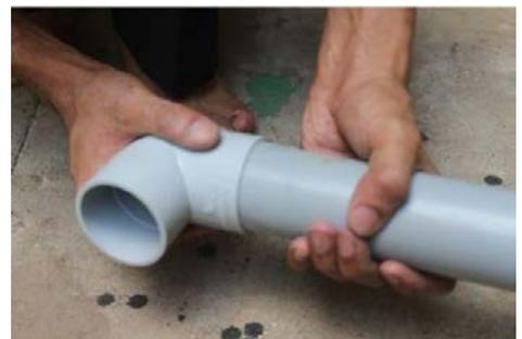
4. Check Pipe placement on the ground, after attaching all Urinals and make sure there is enough space to install the required number of Urinals.
