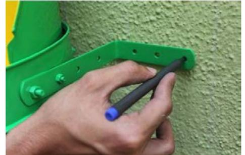
7. Place Urinal against wall again and cross check the marking is matching with mounting holes. Fix the L-angle to the wall using nail and hammer.
