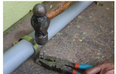
Use a C-clamp to fix the pipe to the ground, where it is loose or is lifted upward.
