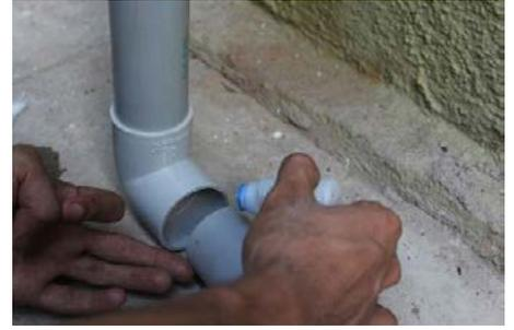
10. Take the strainer and smoothen the edges against a rough surface like wall/floor, so that the strainer side does not have an edge height.
