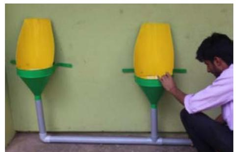
5. Once height of drain pipe and position of Urinal is decided, again ensure there is a small gap between the funnel and the vertical PVC pipe. Hold the Urinal against the wall surface and mark the L-angle holes on both sides.
