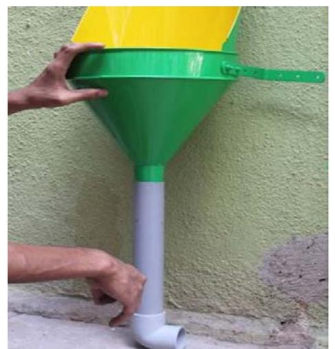
2. Cut the Drain Pipe of 1.5 ft length according to required height with a Hacksaw Blade.
