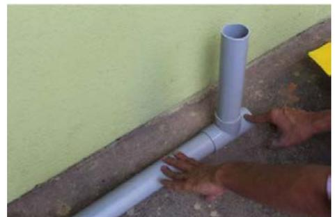
3. The Urinal farthest away from the drain, will have an L-joint to close the piping at that end.
